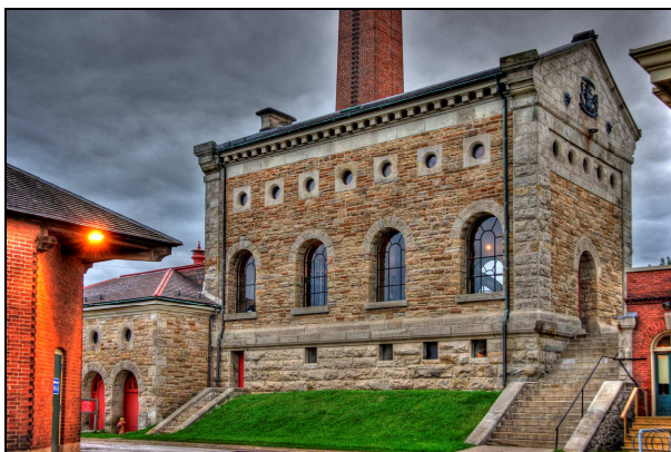
Photo of the c1857 steam-powered pumping station in Hamilton, Ontario, Canada. The engines, which last ran in 1937, are now preserved as a museum. A childhood visit was what began Graham's interest in the water/wastewater sector.
