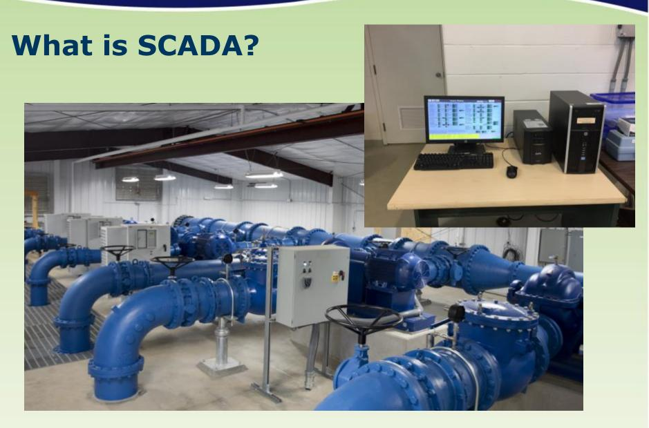
**SCADA = Supervisory Control and Data Acquisition**
