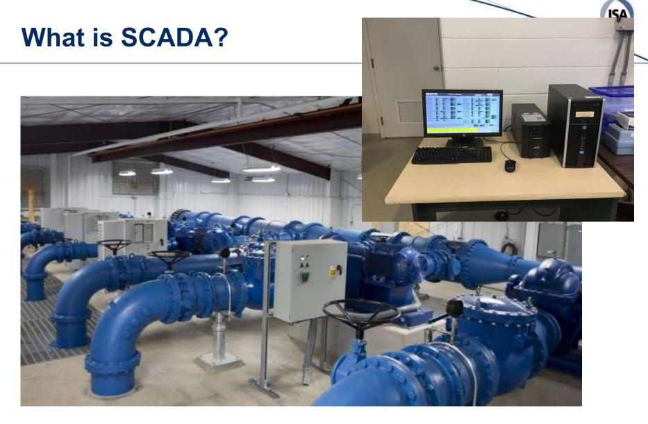
**SCADA** = Supervisory Control and Data Acquisition
